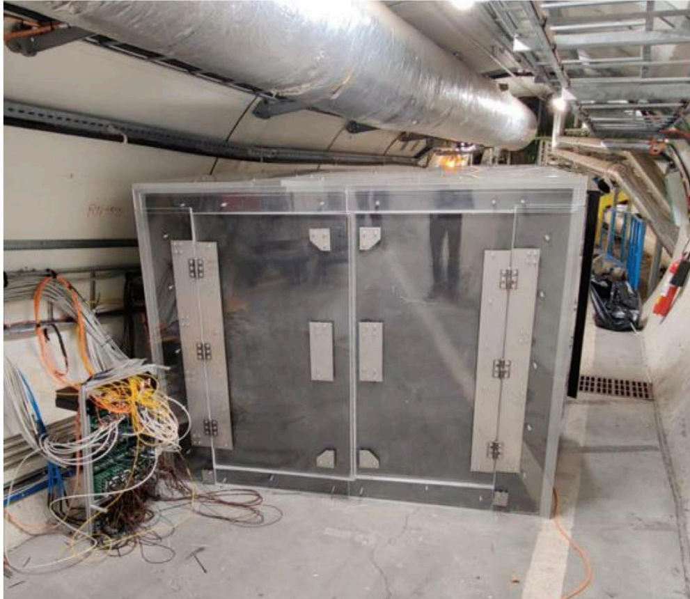
Neutron shield installation: March 2022
