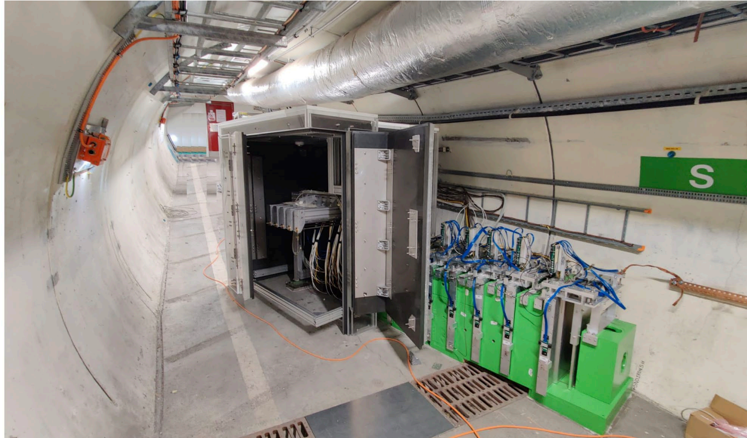
Final completion of the installation: 7 April 2022
